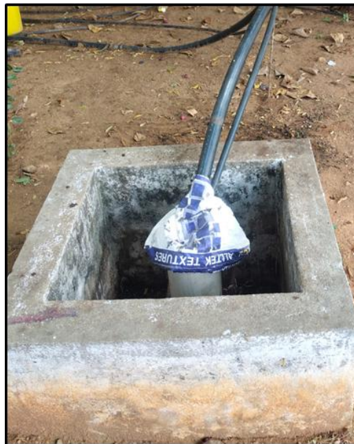
Water Management System observed in the campus
