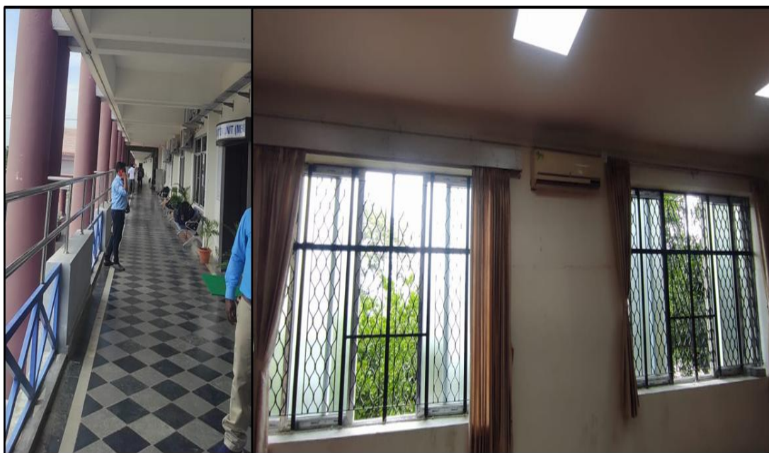
Natural Lighting facilities observed during day time
